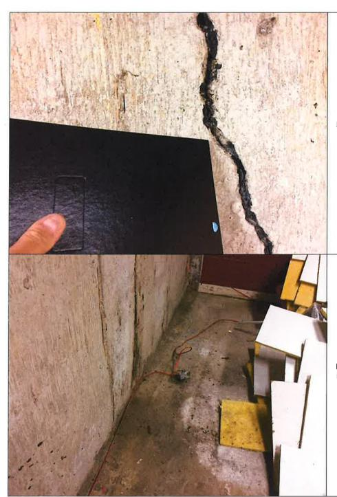
Photo 13: Wide vertical crack in west foundation wall – Note previous attempt to seal crack
