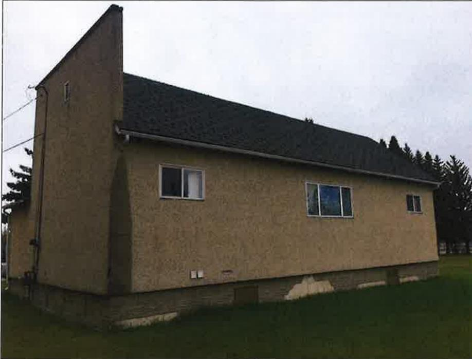
Photo 3: West Elevation – Note missing sections of downspout and water damage to stucco
