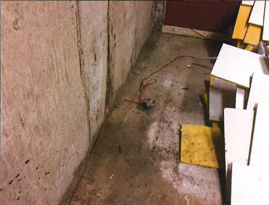
Photo 14: Note signs of water ingress at wide crack in west foundation wall
