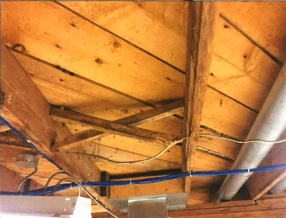
Photo 10: Typical floor joists and decking
