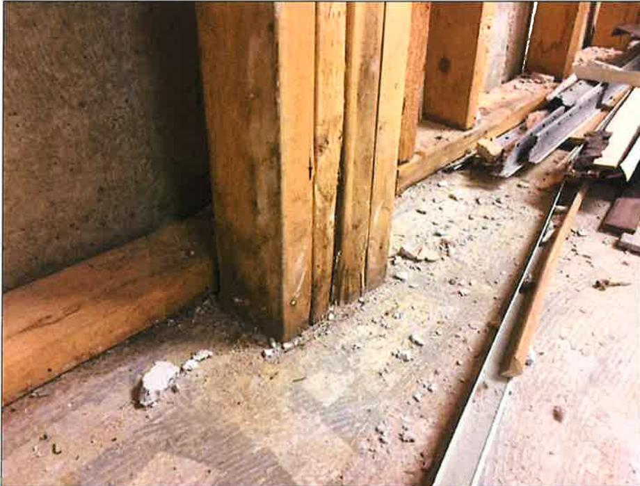
Photo 9: Typical intermediate support beam 4-ply post (bottom connection)
