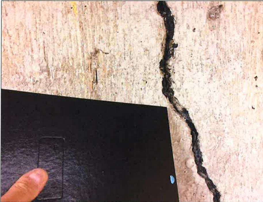
Photo 13: Wide vertical crack in west foundation wall – Note previous attempt to seal crack
