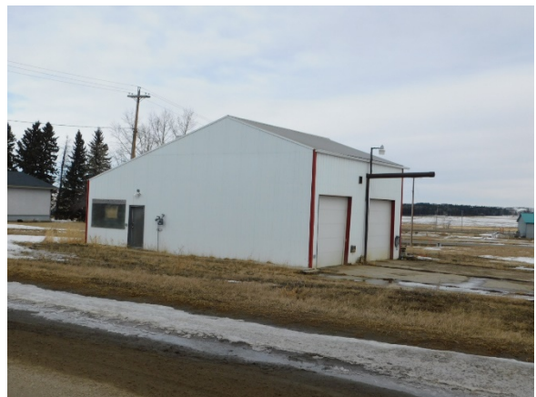
Existing warehouse – assumed removed
